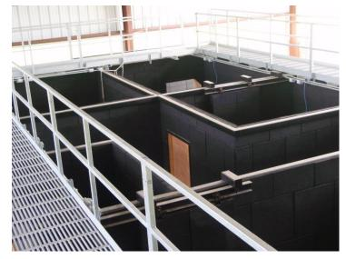
Based upon a legacy of innovative design achievements, Range Systems developed SMASH™, a modular and expandable shoot house that meets the demand for a deployable live-fire training structure. Utilizing standard parts and modular components, SMASH™ offers a balllistically secure shooting facility that is rapidly deployed, requires minimal maintenance, and is adaptable to your training requirements and location.
